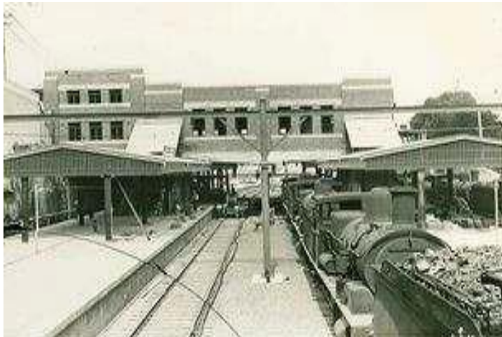
Steam locomotives waiting at North Sydney Station.
