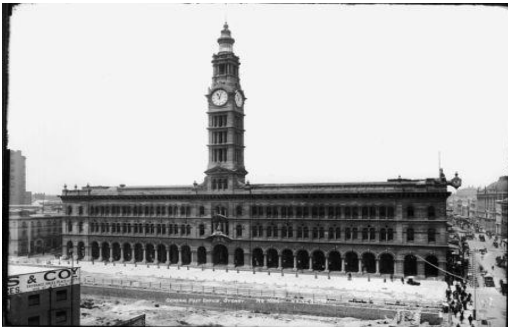
The GPO Clock Tower main façade (circa 1900) located at No. 1 Martin Place.
