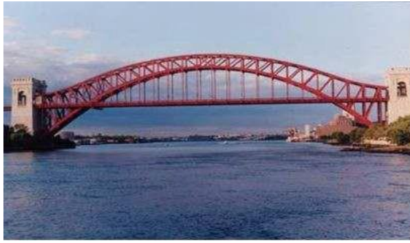
The Hell Gate Bridge of New York, USA first opened on 30 September 1916, spans an impressive length of 310m
