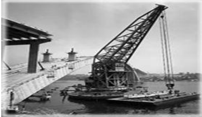
The Gladesville Bridge under construction
